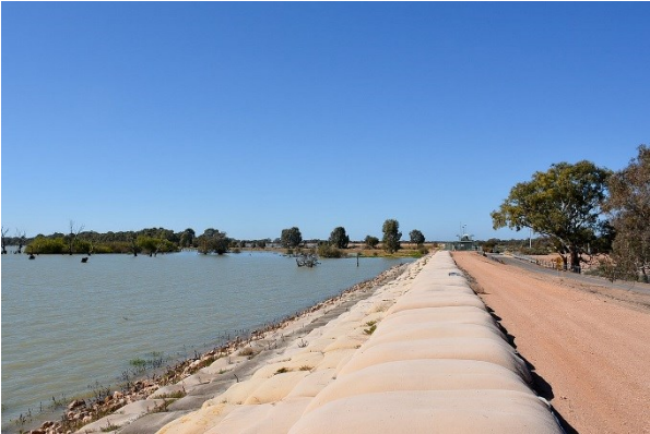
Right: Embankments built to contain lake water. Photos: Murray-Darling Basin Authority
